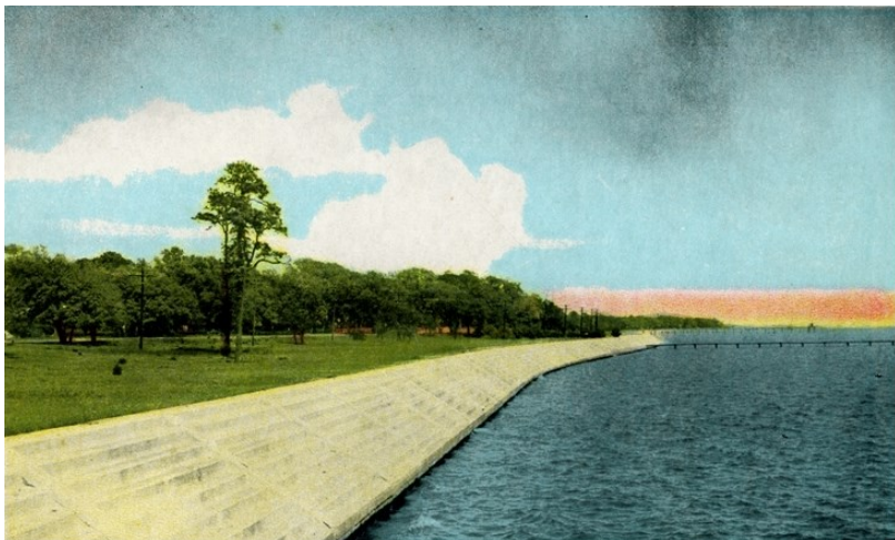
Twenty-six miles of seawall along the Mississippi Gulf Coast (courtesy of MDAH)
